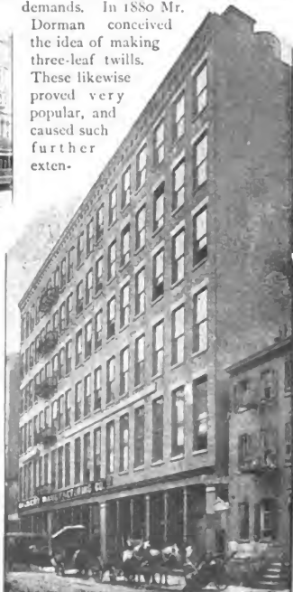
GILBERT MANUFACTURING CO., WAREHOUSE ON CROSBY STREET.
